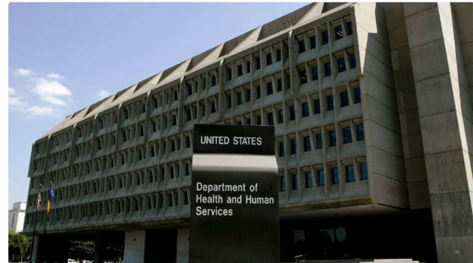
The U.S. Department of Health and Human Services building is shown August 16, 2006 in Washington, DC. Mark Wilson via Getty Images
